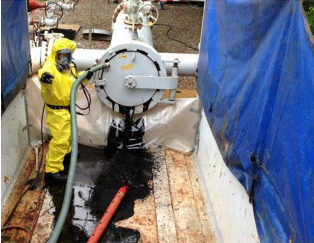
Figure 13. Opening pig receiver.
