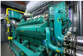
Combined Heat and Power (CHP)
