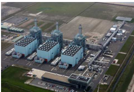
Gas-fired power plants
